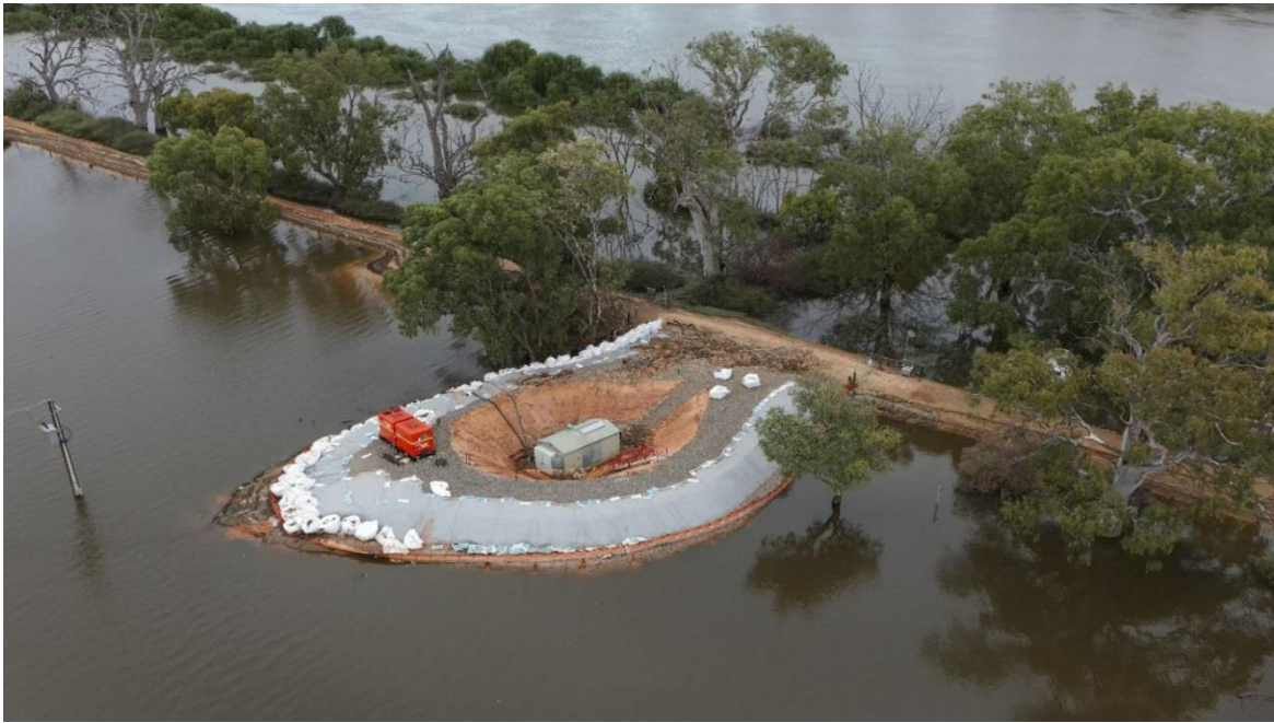
Figure 3-13 Cowirra pump station during flood inundation of adjacent farmland
