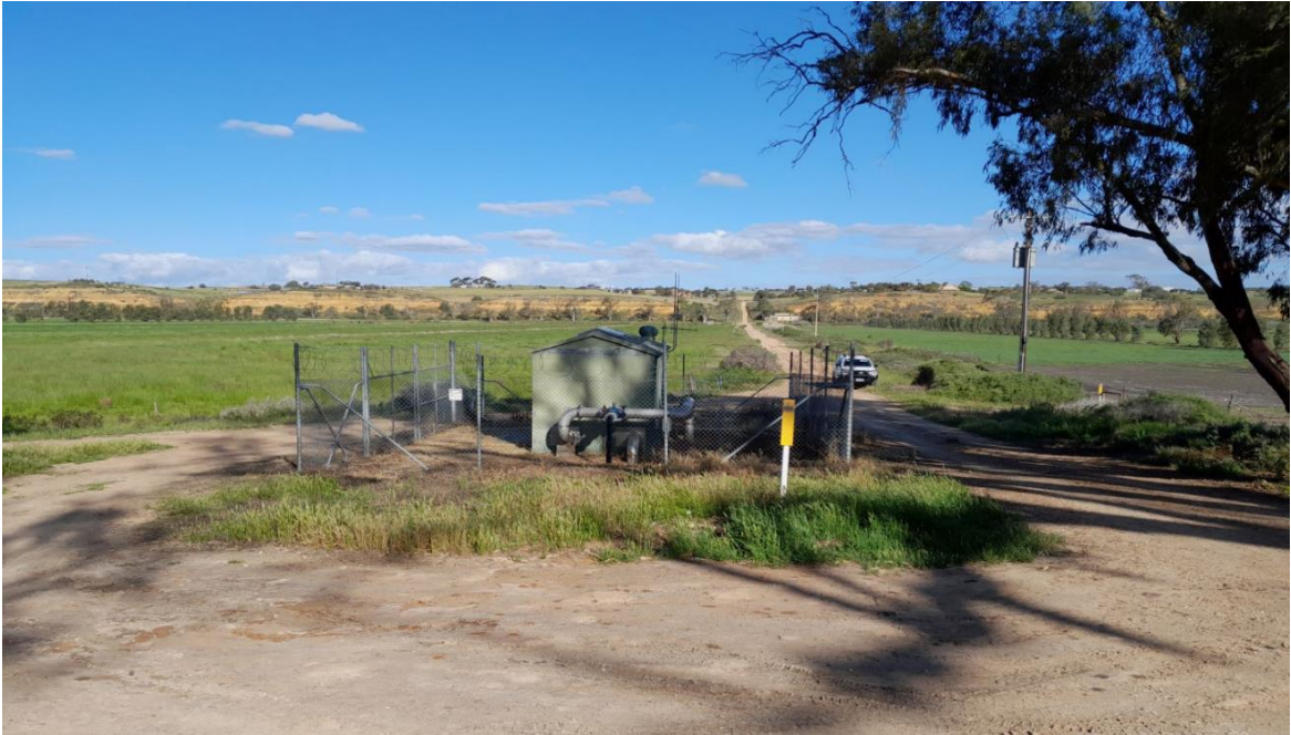
Figure 3-11 Cowirra pump station before levee installation
