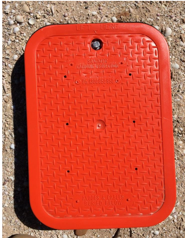
Figure 5-5: A standard anode box. Six breather holes can be seen on the lid.
