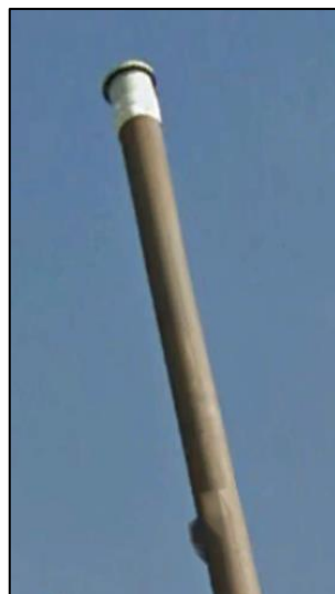
Figure 4-3 Passive AC Filter on Educt
