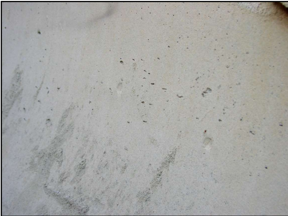
Photo 3: The right side – was vibrated. There has been some “aggregation” of the finely entrained bubbles to give the voids visible in the photograph, but otherwise there is still full contact with the pipe. Vibration is neither necessary nor recommended.
